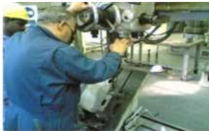
Turbine Body surface works for TSI
