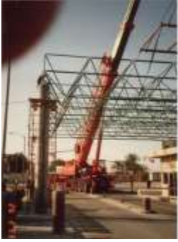
Space frame for Saudi Aramco Station #4
